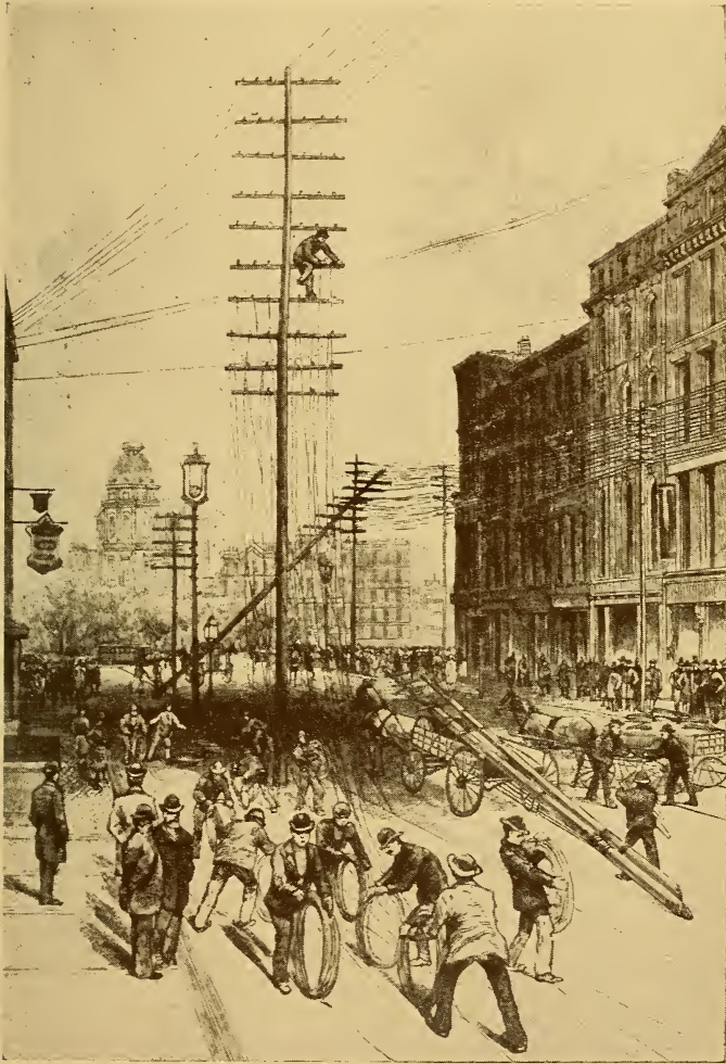
The fight to put telegraph and electric wires underground was a bitter one. Finally, Mayor Grant felled the telegraph pole at the corner of 23rd St. and Broadway with his own hands. The corporations, seeing that he meant business, succumbed to the inevitable.
